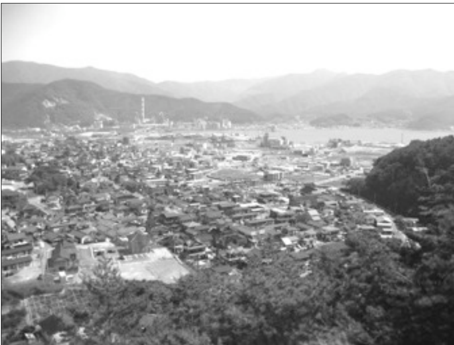
Ofunato, one of the disaster-stricken towns in Iwate
