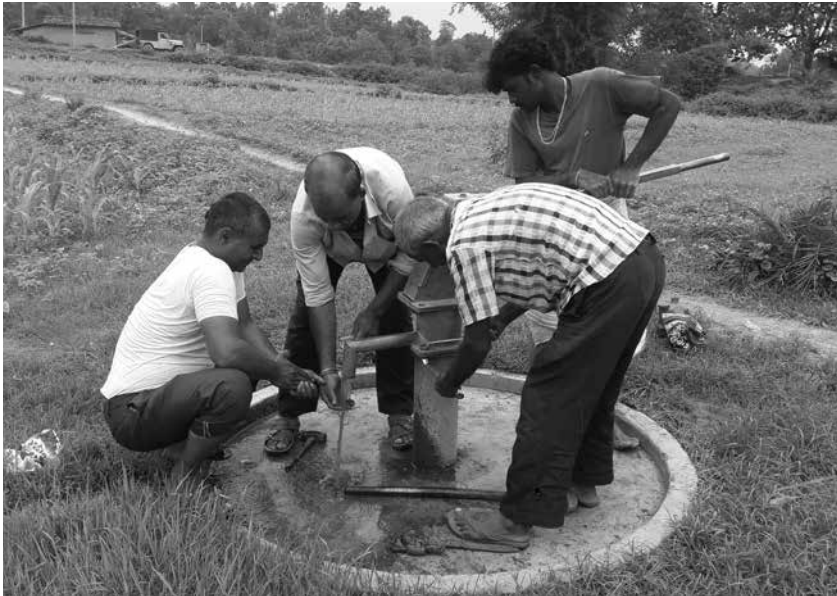
Repairing handpumps by the community to ensure safe drinking water supply.
